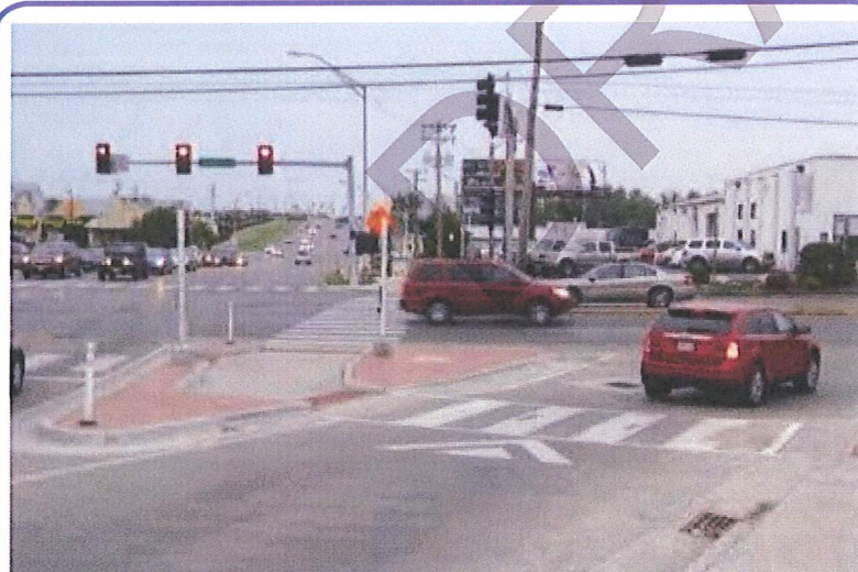
Channelized Raised Crossing (Columbia, Montana)
